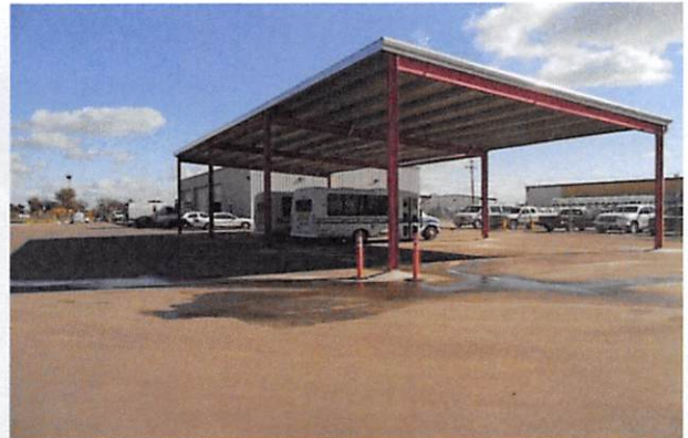
Asphalt of corporate yard and bus shelter
